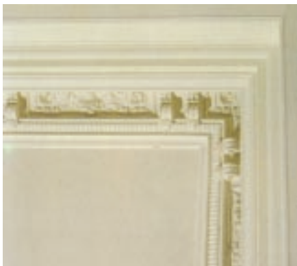
Stuccoed ceiling in the northeast wing
