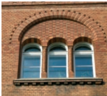
Triplet windows with checkerboard pattern
